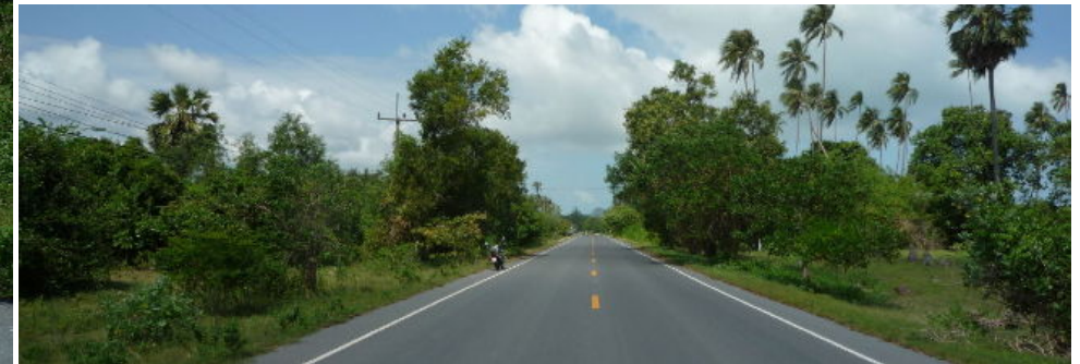
bottom right: view to the north
